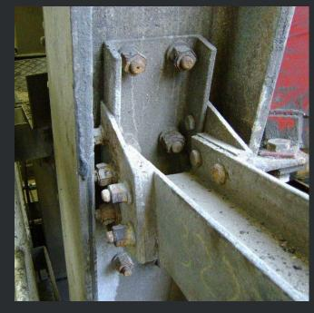
Bolted joints require regular inspection.
