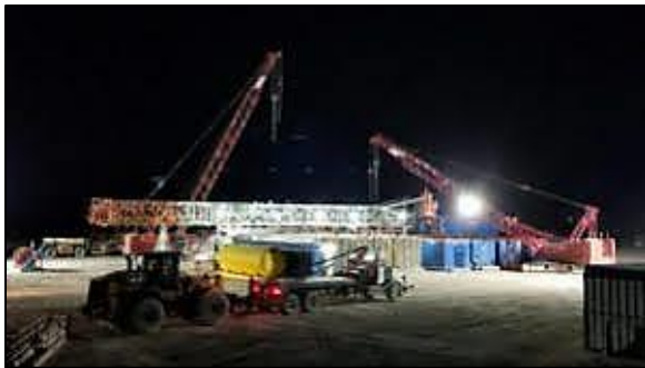
Figure 1 - Rig Move Night Operations
