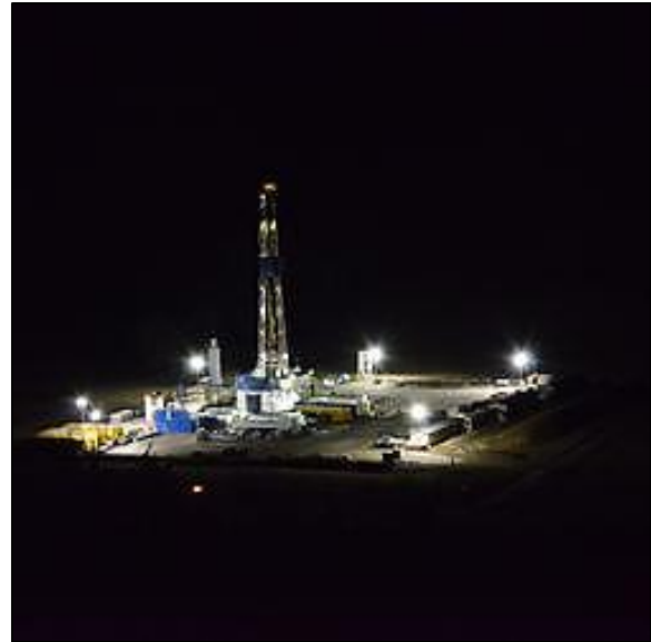
Figure 2 - Rig Pad Site with Light Plants
