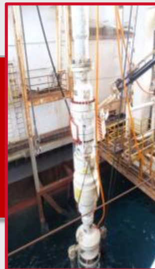
Integrated RCD (DP) Below Tensioner Ring
