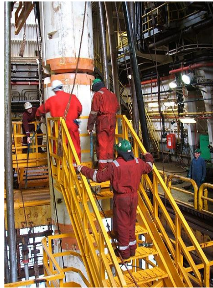
Above: Running riser with safe access to umbilical clamps hoses etc.
