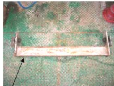
Stopper plate not in position
