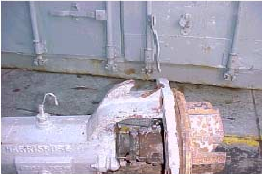
Location of Integral Lifting Eye Failure
