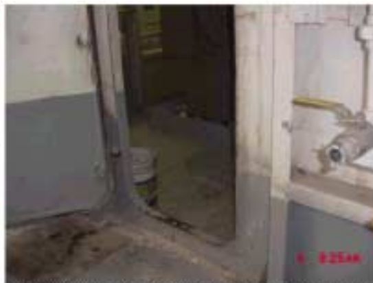
Figure 2: The watertight door that they set the rod down on.
