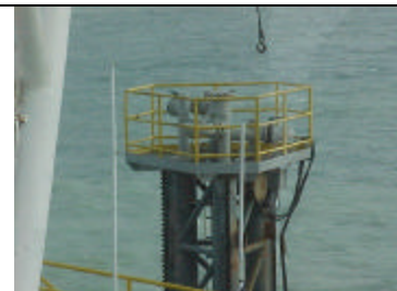
#2 Crane Operator's view of Deep Well Tower
