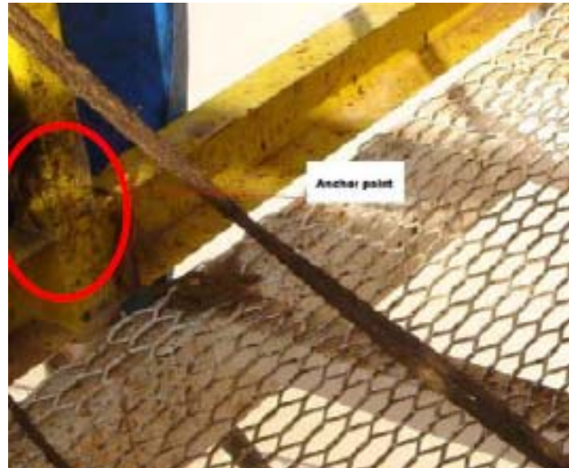
Point of attachment on handrail.
