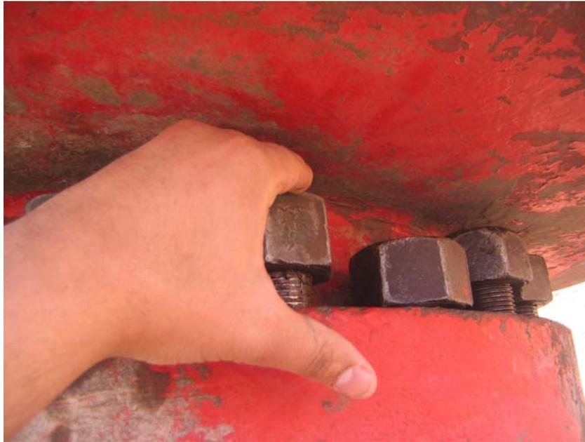
The pinch point area between the annular body and the BOP bolt where the IP placed his left hand fingers.
