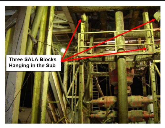
The scaffolding is a floating design. The walkways are scoped up or down on tracks on the four corners.
