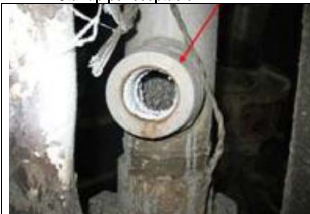
Standpipe receptacle
