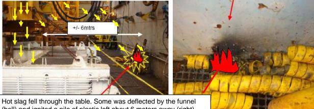
(bell) and ignited a pile of plastic left about 6 meters away (right). The fire was immediately extinguished.
