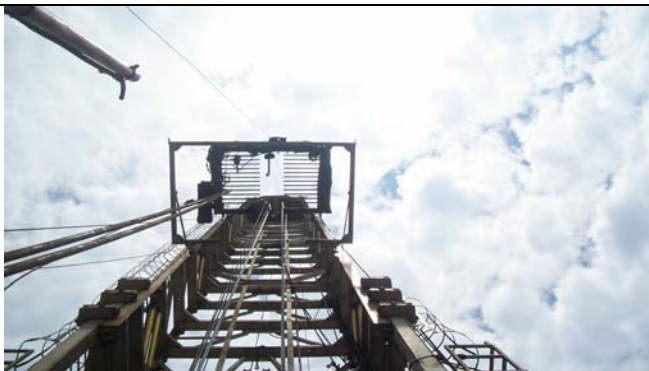
View of missing diving board
