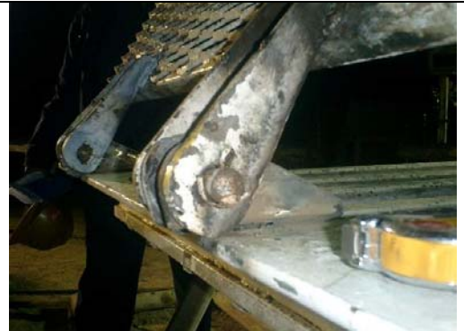
Re-enactment of backside of pad eye rubbing at 45 deg angle. Actual restriction was on Monkey board beam.
