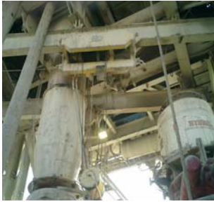
Figure 1 – Overhead Crane Set-up
